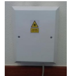
Wall-mount Fiber-to-Home Optical Node (ONU-Mini_1)
